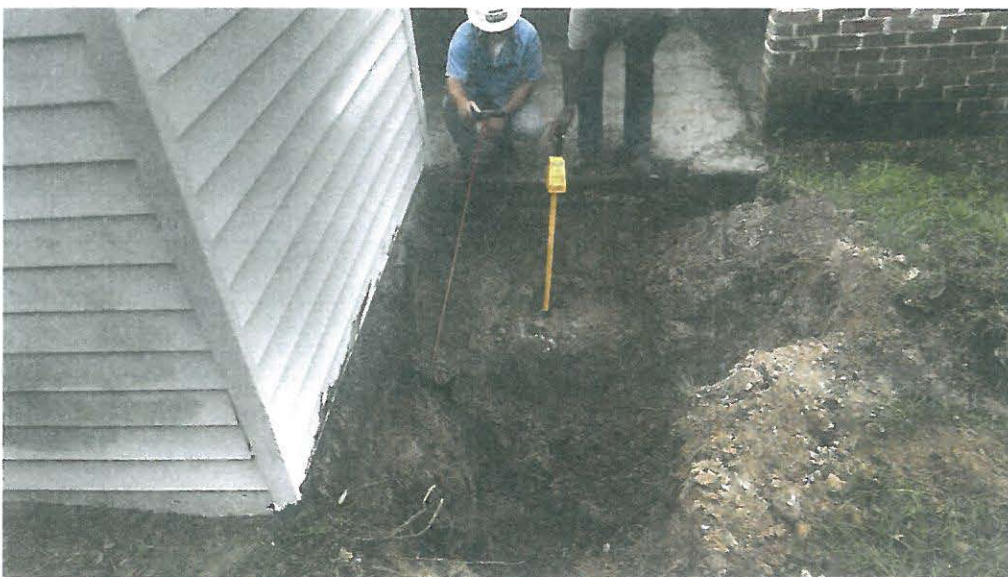
Picture 2: UST 1184Bobwhite excavation in progress. Workers are pointing to the buried tanks.
